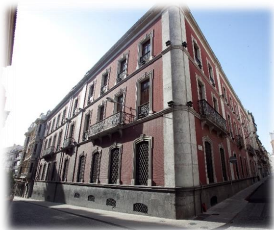
Edificio García Lovera (Córdoba) Hotel currently under refurbishment
