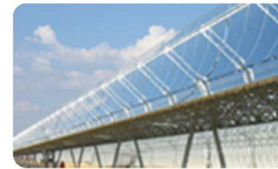
Parabolic Trough - Solnova 1
