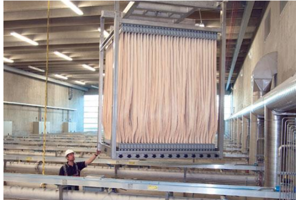
Worker installing hollow fiber membranes in MBR
