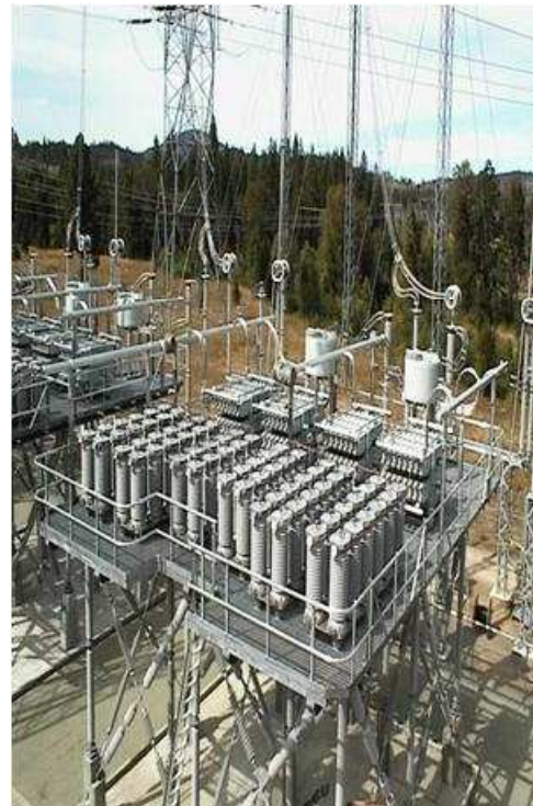
Example of series compensation planned for Anglo Scottish Interconnector allowing additional 1GW of capacity
