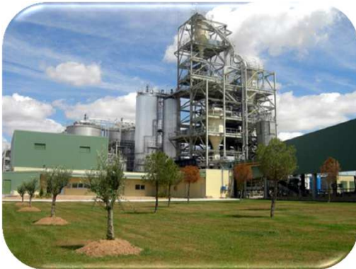
Cellulosic ethanol demonstration plant (5 ML/yr) in Salamanca (Spain)
