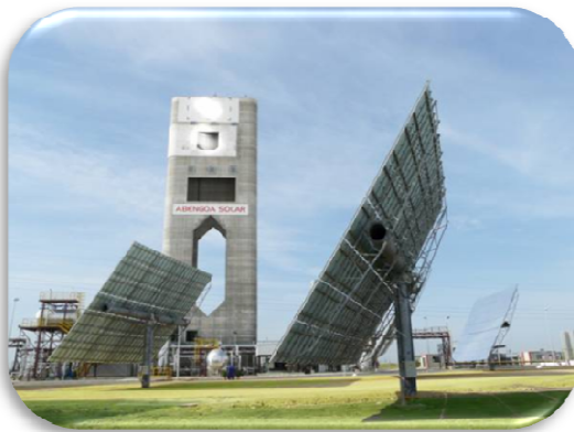
Superheated steam “Eureka” pilot plant
