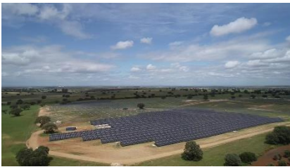
Alvarado (100 MW) Build & Sell - Spain
