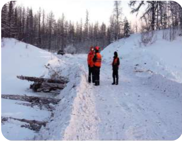
Building of a crossing over the river.
