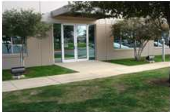
Austin Testing Laboratory, TX
