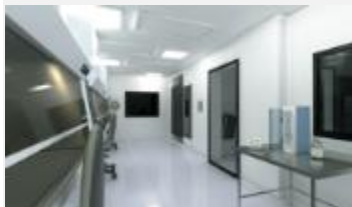
Compliant sterile cleanrooms
