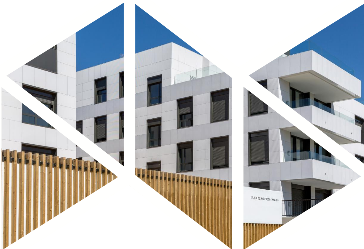
AIGUADOLÇ HOMES – SITGES (EAST REGION) Actual picture (June 2019)
