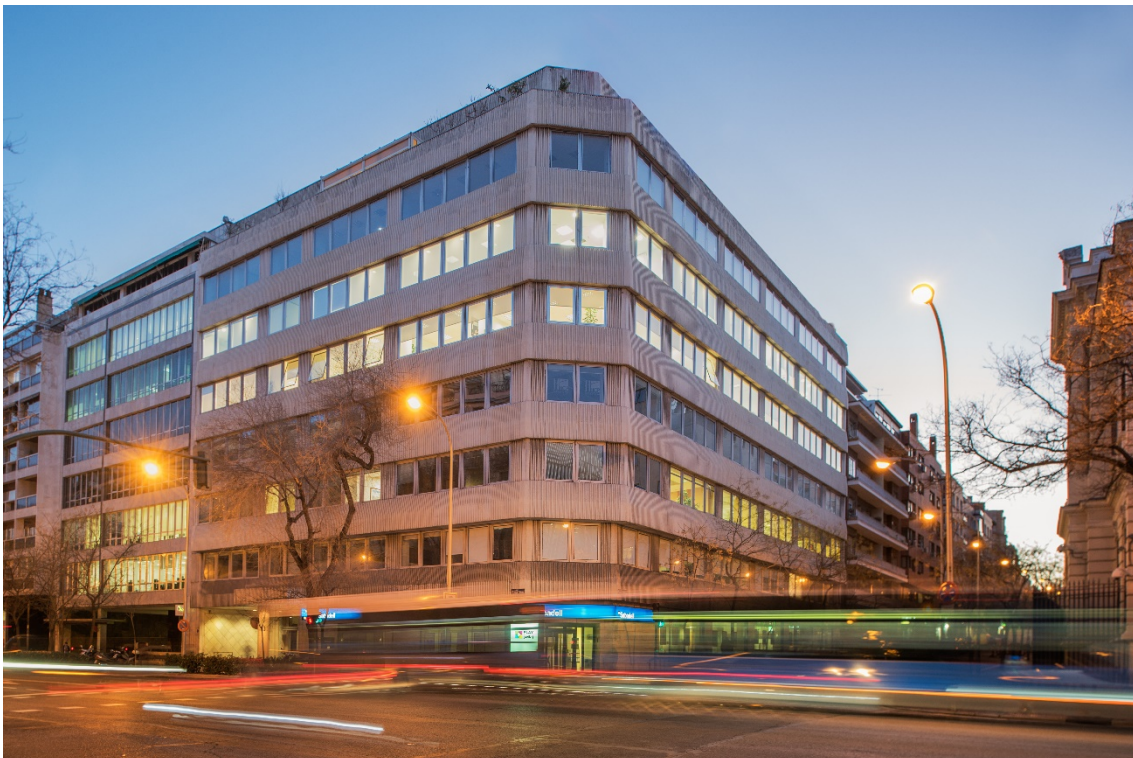
Photo: Axiare Patrimonio. Building on Calle Miguel Ángel, 23
