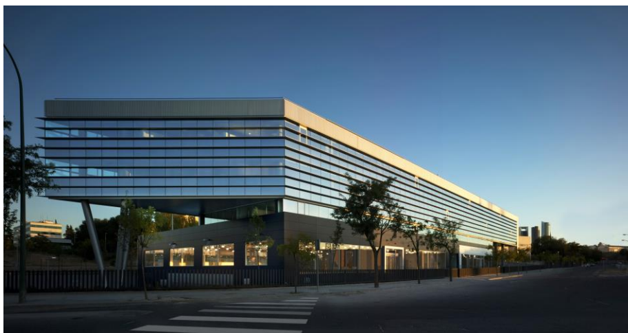
Photo: Puerto de Somport 8 Building, Madrid, owned by Axiare Patrimonio
