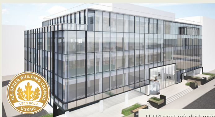
JILT14 post refurbishment
