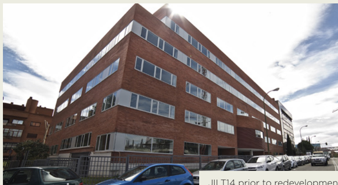
JILT14 prior to redevelopment
