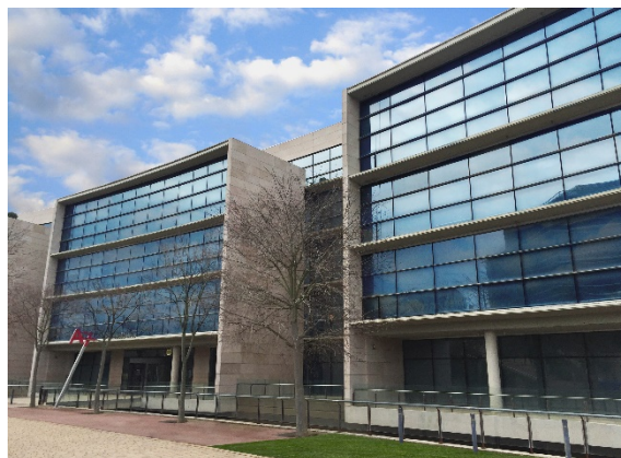
Photo: Axiare Patrimonio. Building located on Avenida Can Fatjó dels Aurons
