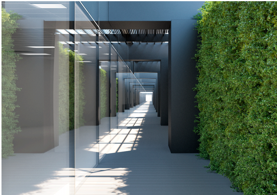
Photograph: Axiare Patrimonio. Lower ground-floor of the Manuel de Falla building in Madrid.
