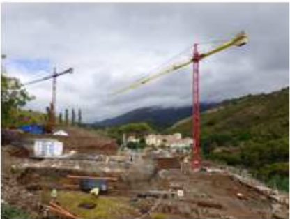
WIP Quabit Riverside. Málaga 75 Home units
