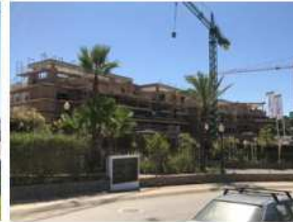
WIP Quabit Casares Golf 1 y 2. Málaga 87 Home units
