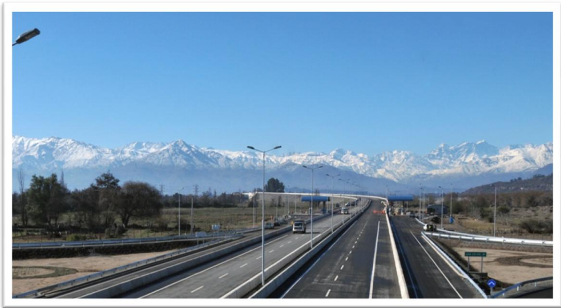
Toll roads – Chile
