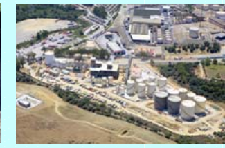
San Roque, Sp 250 MI/year Construction
