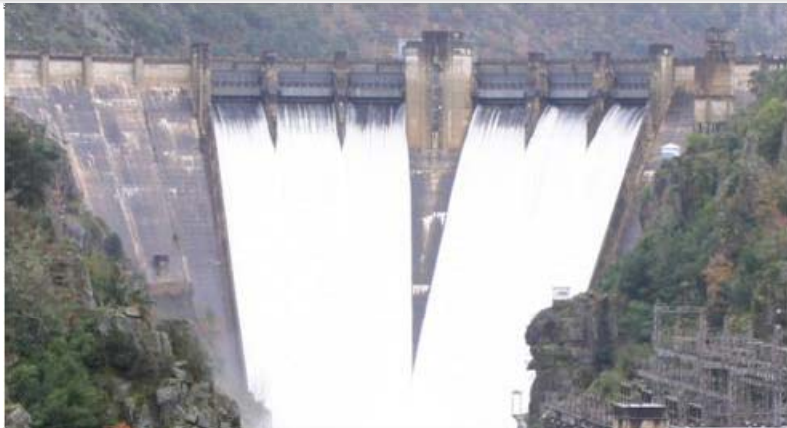
CH San Esteban II, 175 MW Operating in 2012
