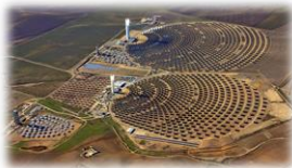
Solucar Platform Solar (Seville, Spain)
