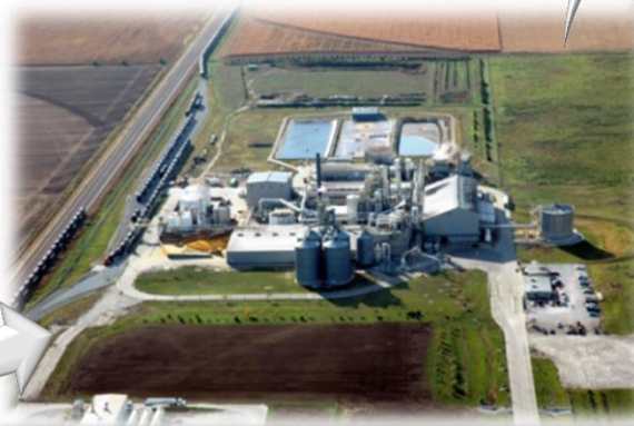
Pilot Plant York
