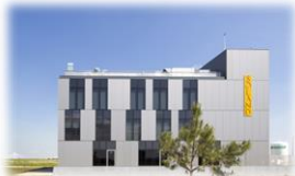
Soland R&D Center Solar (Seville, Spain)
