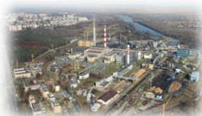
Stalowa Wola (Poland) Combined Cycle 450 MW
