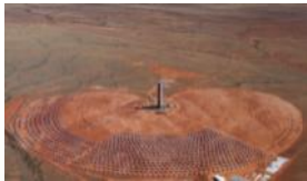
Superheated steam tower
