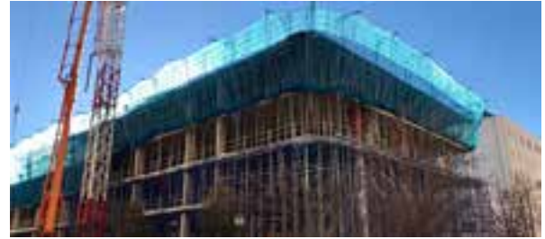
Lagasca 99 Building works (Madrid)
