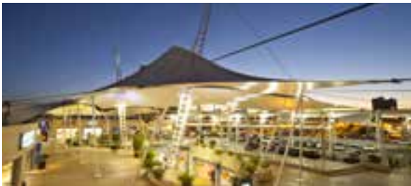
Vistahermosa Shopping Centre new image (Alicante)
