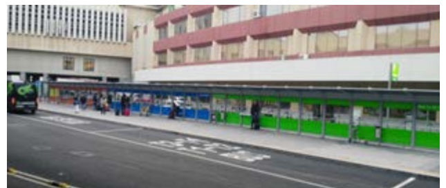
Figure 15. Road access. A.S. Madrid-Barajas Airport
