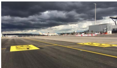
Figure 16. Taxiway paving repair. A.S. Madrid-Barajas Airport
