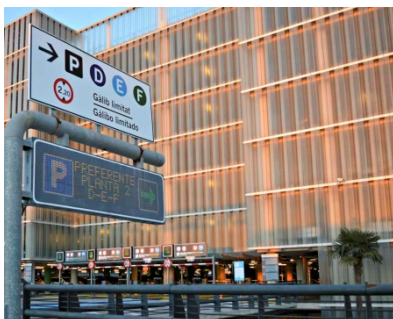
Figure 28. Parking. Barcelona-El Prat Airport
