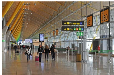
Figure 1. Terminal T4 – Adolfo Suarez Madrid-Barajas Airport
