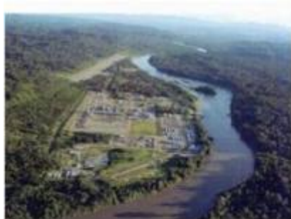
UPSTREAM (Exploration & Production)
