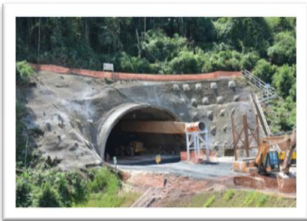
Duplication of Serra do Cafezal (Régis Bittencourt toll road)
