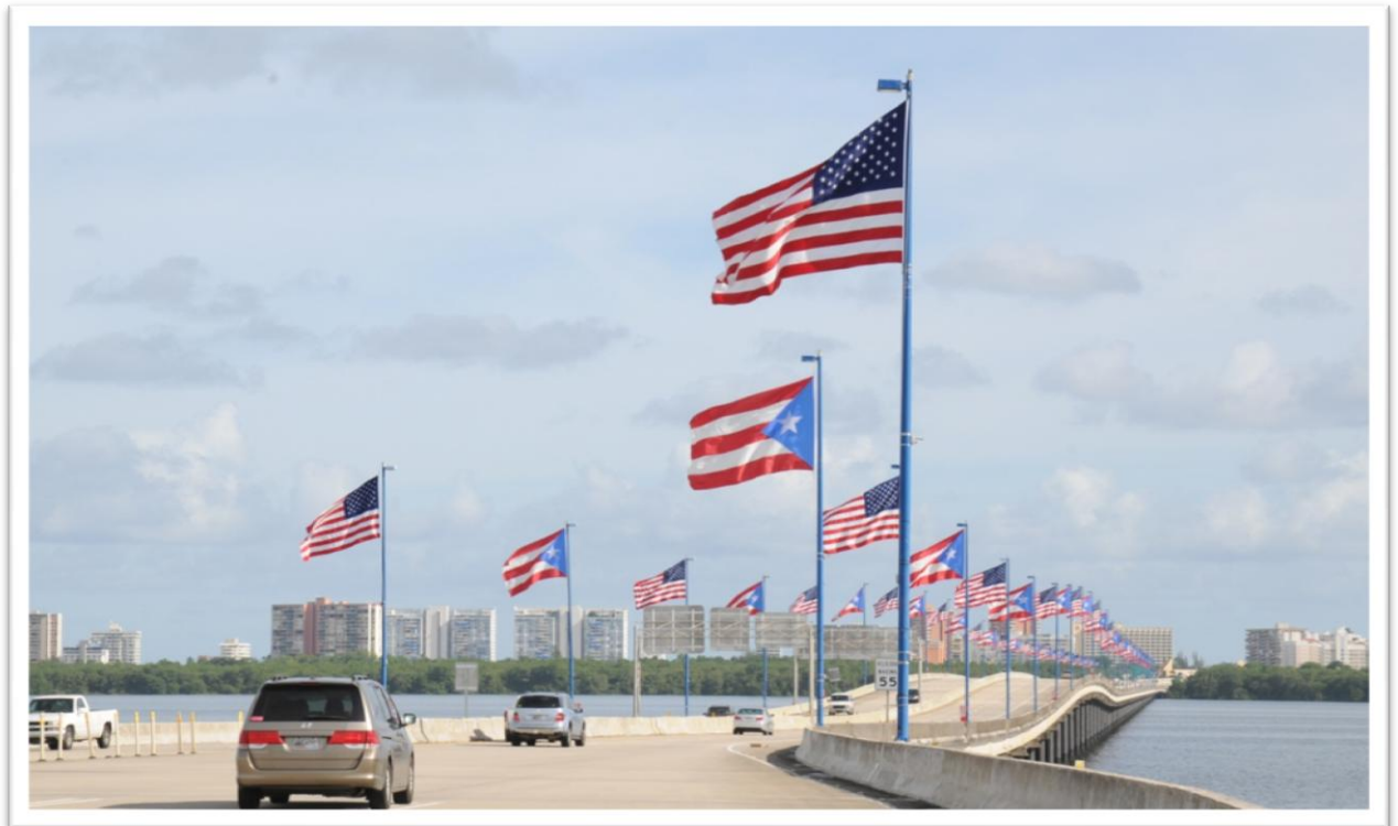
Teodoro Moscoso Bridge- Puerto Rico
