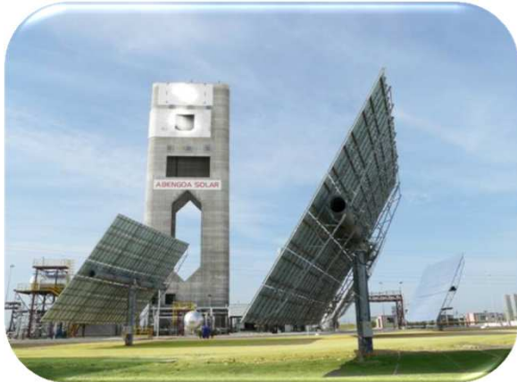
Superheated steam »Eureka« pilot plant
