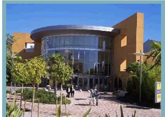
Tres Aguas: 65.130 m 2 (C. C.)
