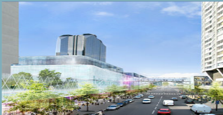
Beaugrenelle center: 13.004 m 2
