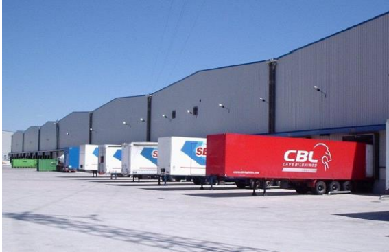
Outside View of Logistics Platform
