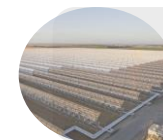
50 Mw Puertollano Thermosolar plant
