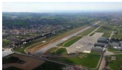
Picture 18. Runway refurbishment. Son Bonet Airport
