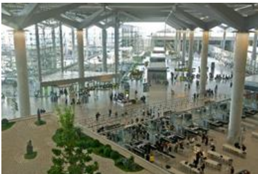
Picture 5. Inside the terminal - Málaga-Costa del Sol Airport
