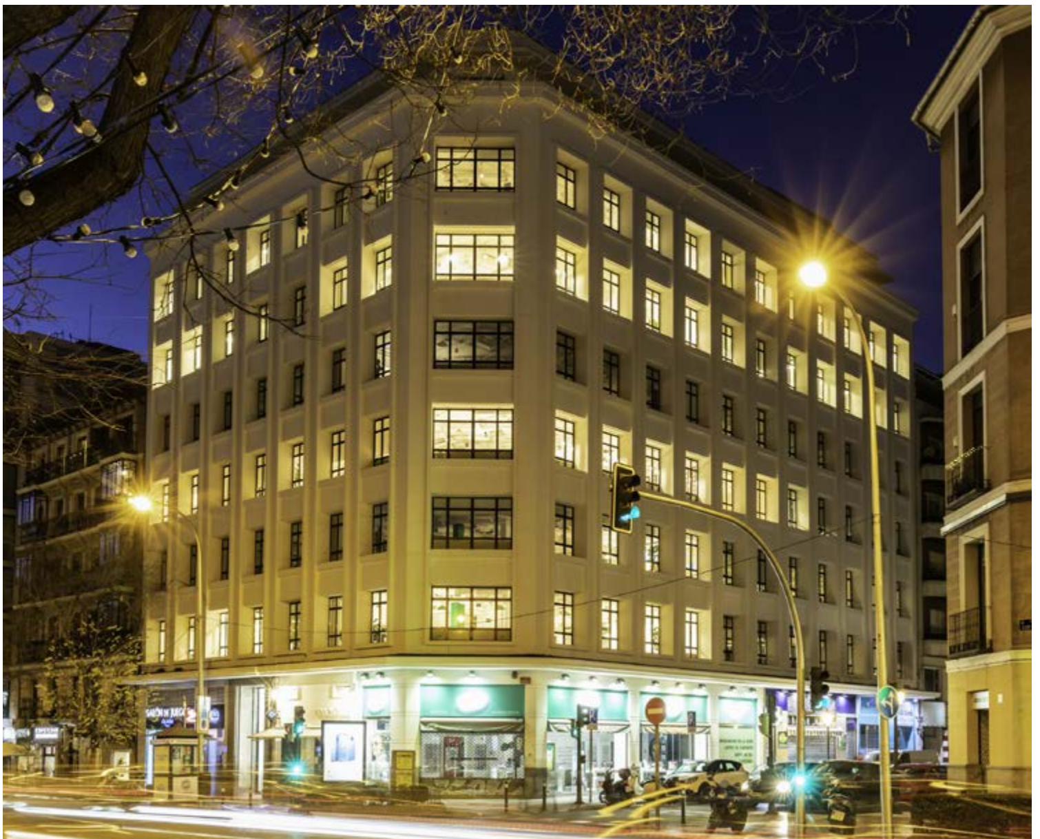
Eloy Gonzalo Office Building (Madrid)
