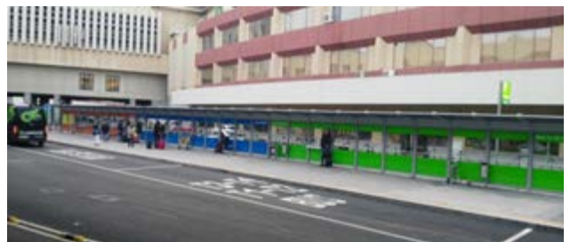
Figure 15. Road access. A.S. Madrid-Barajas Airport
