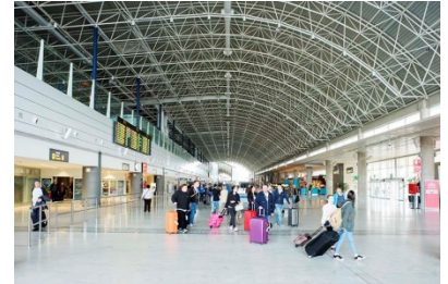
Figure 4. Fuerteventura Airport terminal
