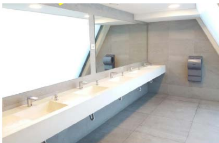
Figure 11. Refurbishment and modernisation of lavatory facilities. Bilbao Airport
