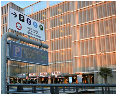
Figure 28. Parking. Barcelona-El Prat Airport
