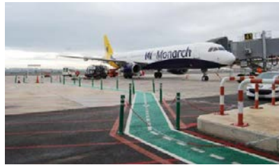
Figure 17. Modernisation of pedestrian pathways. Alicante-Elche Airport
