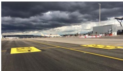
Figure 16. Taxiway paving repair. A.S. Madrid-Barajas Airport
