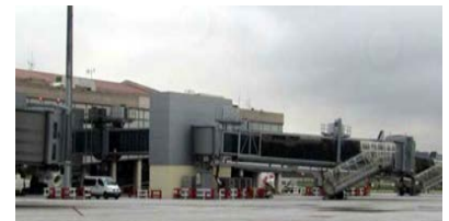
Figure 21. New air bridges. Málaga-Costa del Sol Airport
