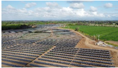
Quinantu (12 MW) Build & Sell - Chile
