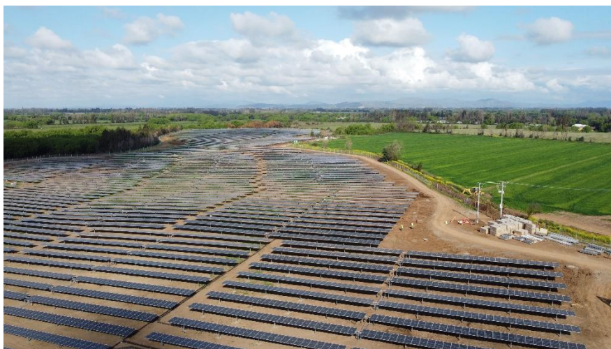
Quinantu plant under construction in Chile
