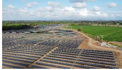
Quinantu (12 MW) Build & Sell - Chile
