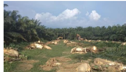
3SP (116 MW) Build & Own - Malasia
