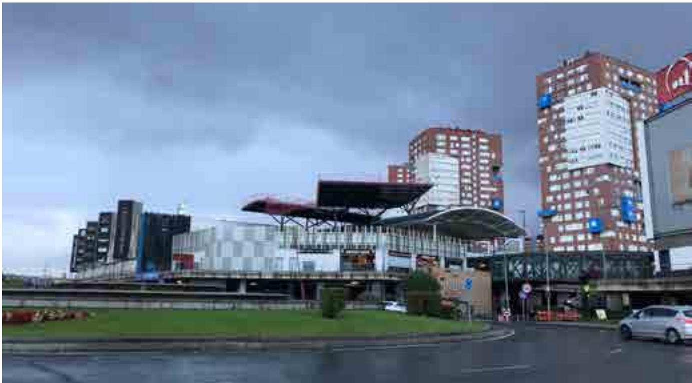
Megapark retail park (Barakaldo) after the completion of part of the refurbishment works.
