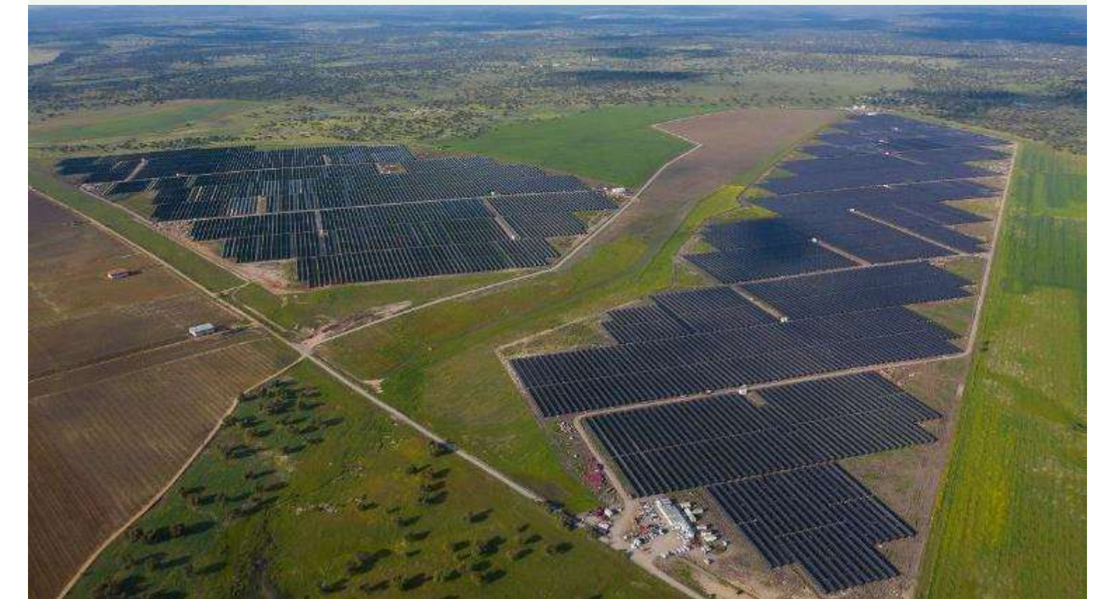
100MW photovoltaic project in Spain
