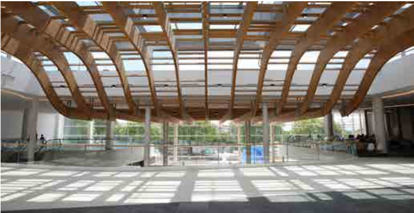
Ànec Blau shopping centre (Barcelona) after the completion of part of the refurbishment works.
