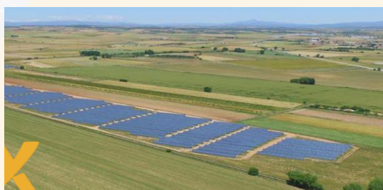
PV Cañamares (Guadalajara) 5 MWp
