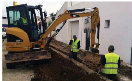
Construction of gas network – Portugal 16M€ - In execution
