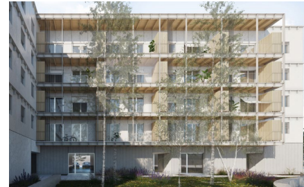
Social housing – Navarre, Spain. 5M€ - In execution
