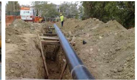
Construction of gas network – Faro, Portugal 1M€
