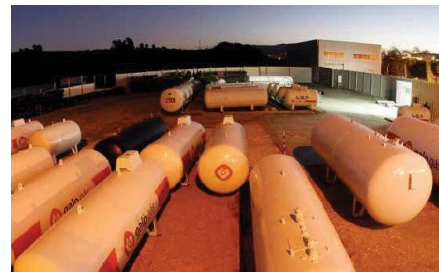
Refurbishment of lpg tanks – Portugal 800K€
