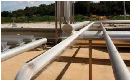
Construction gas network – Portugal 450K€
