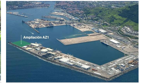
Extension of Pier AZ-1 – Bilbao, Spain 27M€ - In execution
