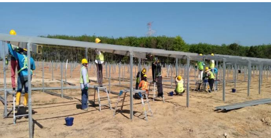
3SP plant Under Construction in Malaysia
