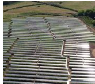
Quinantu 12 MW Build & Sell Chile
