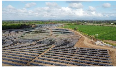
Quinantu (12 MW) Build & Sell - Chile
