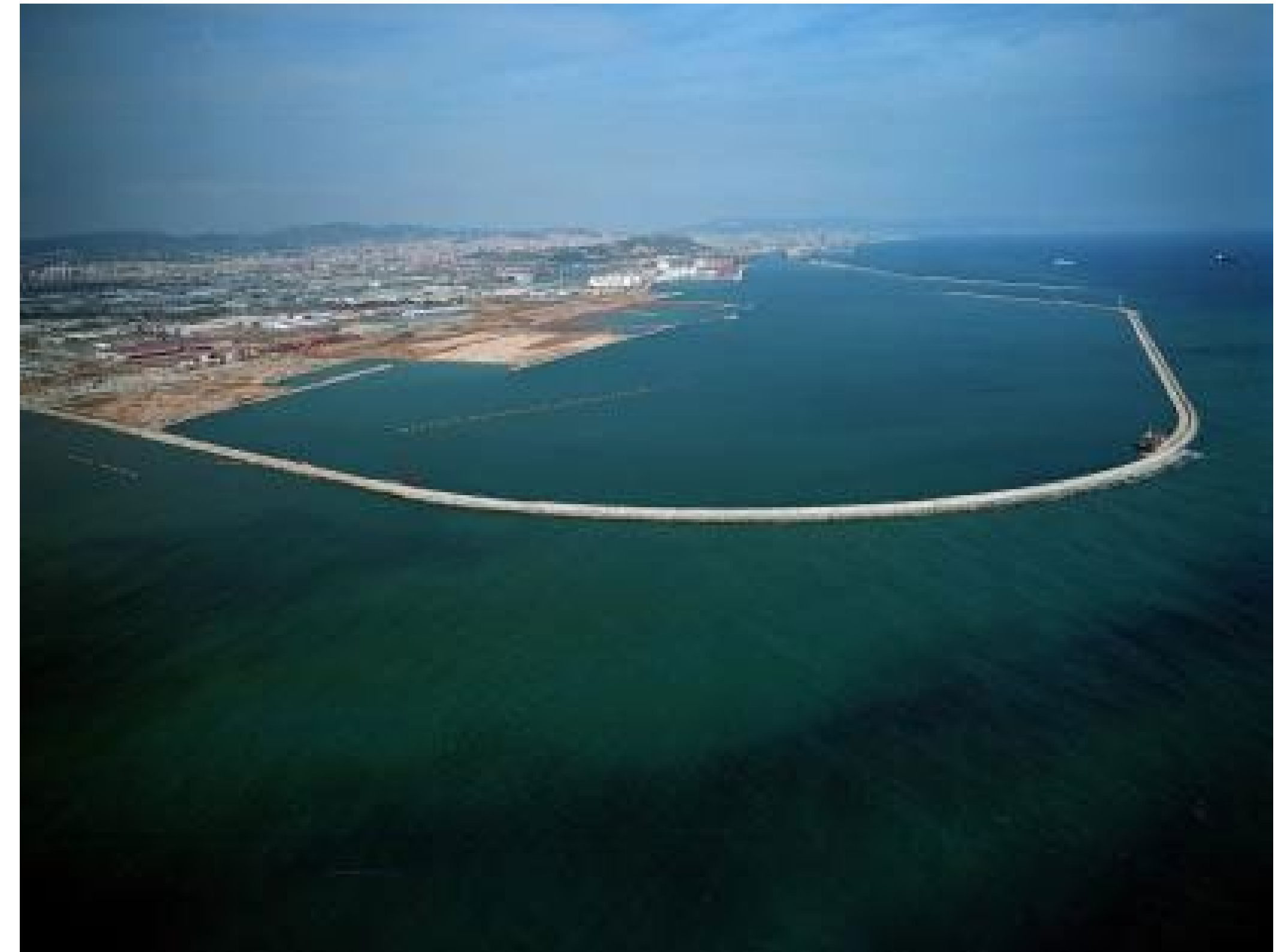
Southern Barrier Tranche I, II and III, Port of Barcelona, Spain.
