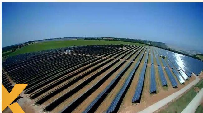
PV Carolinas (Guadalajara) 10 MWp
