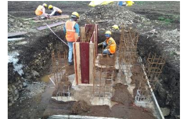
KA2-AFZ (28 MW) Build & Own - India
