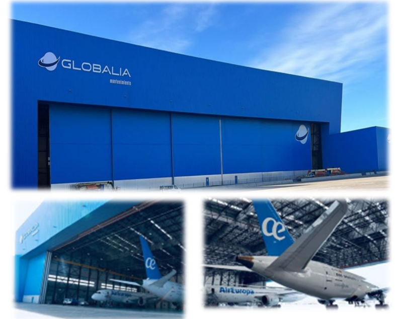
New Globalia maintenance hangar at Adolfo Suárez Madrid-Barajas Airport
