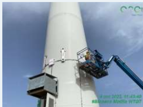
Installation of bird protection system at Motilla wind farm
