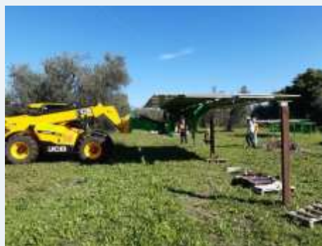
Pre-assembled system installation test
