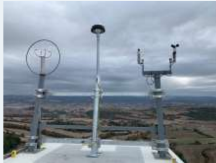
Lightning protection system in wind turbines
