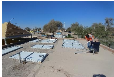
Rooftop installation in a school near Pozo Almonte
