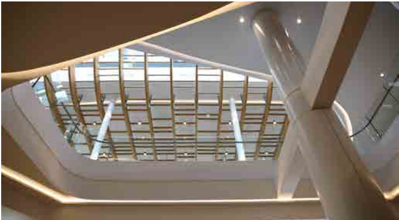
Shopping Centre Ànec Blau (Barcelona) after the completion of part of the refurbishment works.
