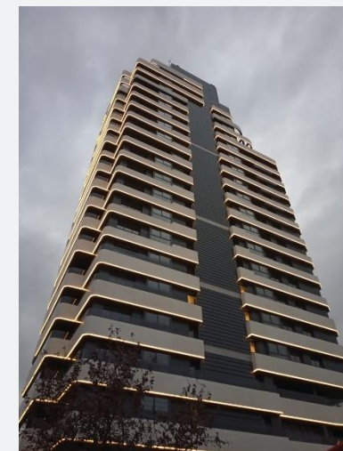
RIVERSIDE HOMES – CENTER REGION
