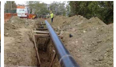
Construction of gas network – Faro, Portugal 1M€
