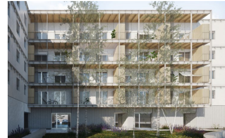
Social housing – Navarre, Spain. 5M€ - In execution
